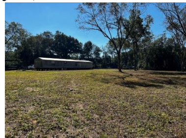
This is the mobile home where the septic tank was installed.
